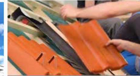
FINISHING WORKS IN CONSTRUCTION
